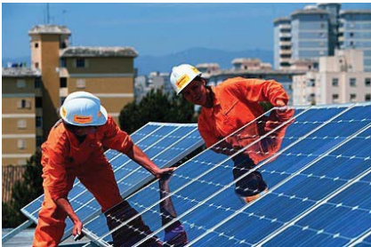
Figure 1. Installation of silicon based solar cells onto a roof
